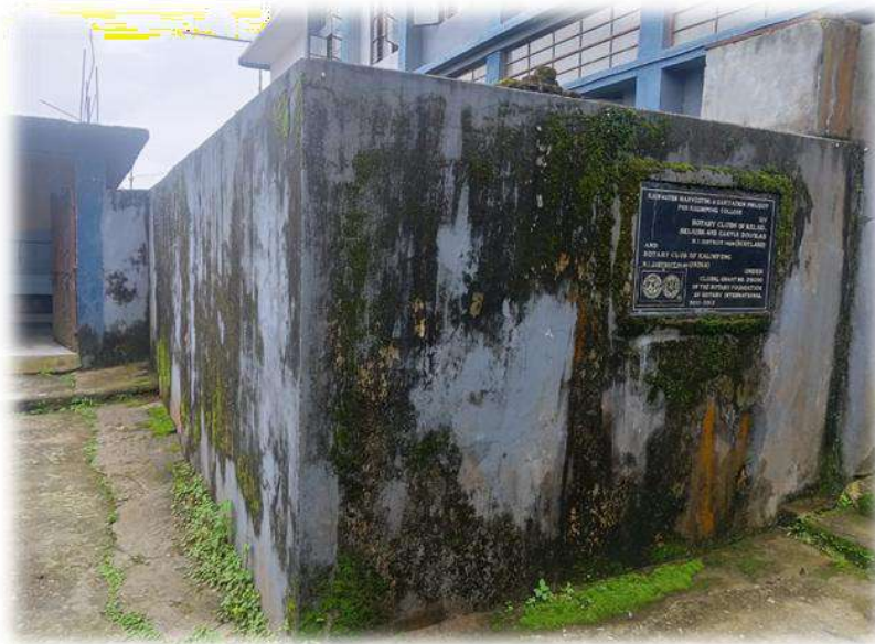
1, 64, 000 liters water harvesting tank at College Campus (Sufficient quantity for the College campus)
